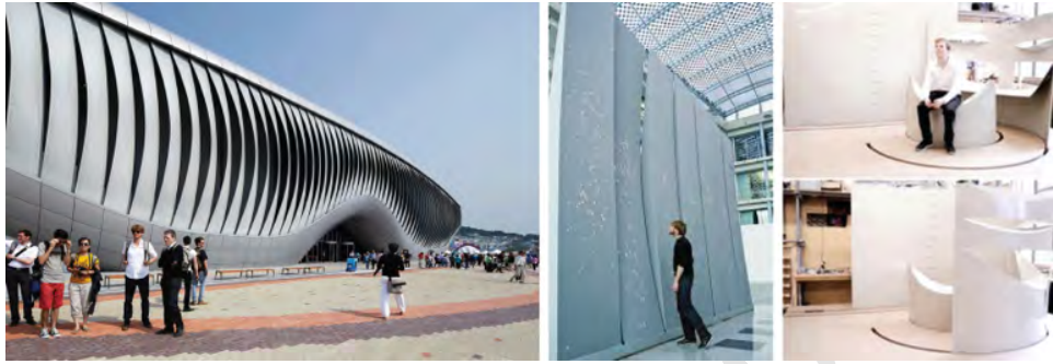
Figure 3.12 Left: One Ocean Pavilion, designed by Soma Architecture [som] and created for the South Korea’s Expo in 2012, has a kinetic facade with slats that open and close individually to create a rippling effect (photo Soma Architecture). Middle: The Hyperbody group develops prototypes to explore the possibilities of computationally driven interactive architecture based on swarm theory. The large panels can move based on external conditions forming a movable wall (Photo by Festo AG). Right: The Hyperbody group creates also shape-shaping interior and furniture (Photo taken by Hyperbody TU Delft).
