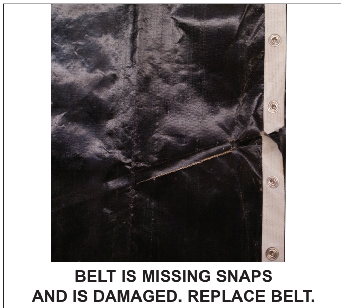
Figure 6. Example of Damaged Belt
