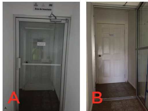
Figure 15. Examples of safety vestibules with double doors
