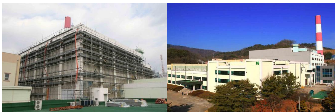
Figure 3. HANARO during and after seismic reinforcement construction
