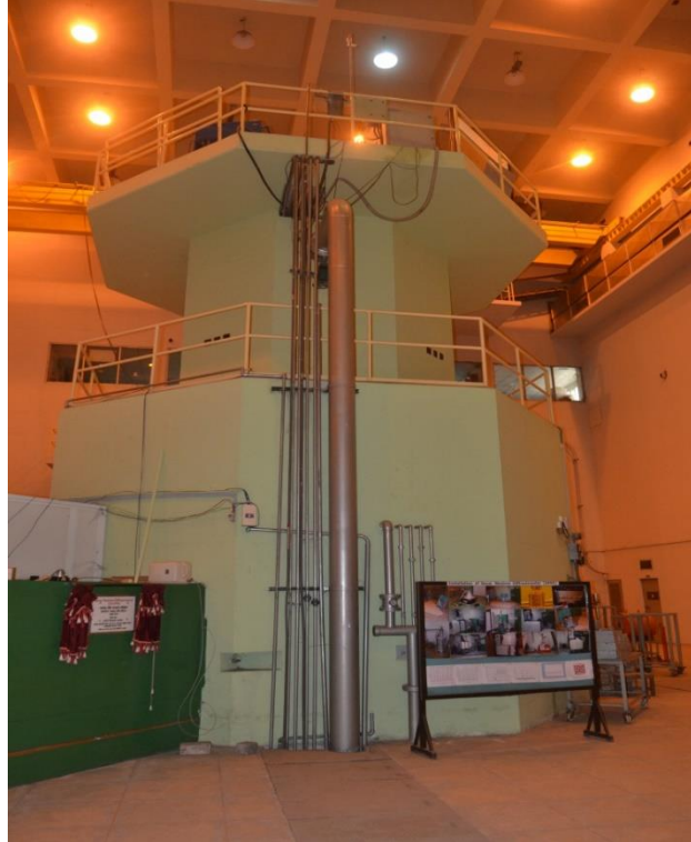
FIG.1. Shield structure of the BTRR
