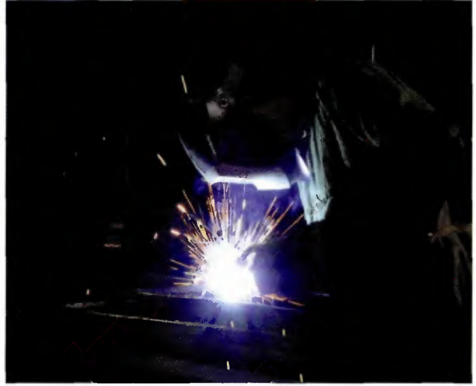
Fig. 3 — Employee Joshua Neumayer gas metal arc welds steel rails.
