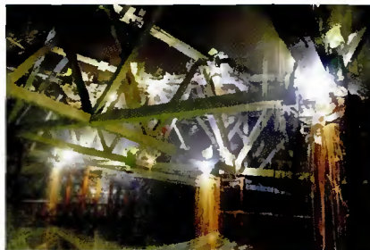
Workers finish welding the steel structure of the Bird's Nest.
