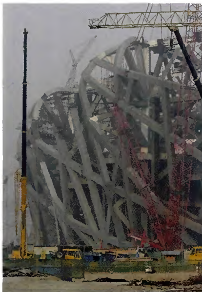
The supporting structures awaiting removal.
