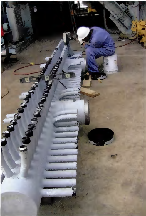
Fig. 1 — The 15-ft header is prepped for welding.
