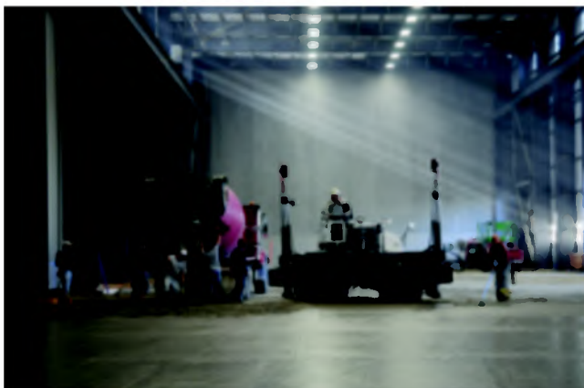
The new building comes together during its construction phase.
