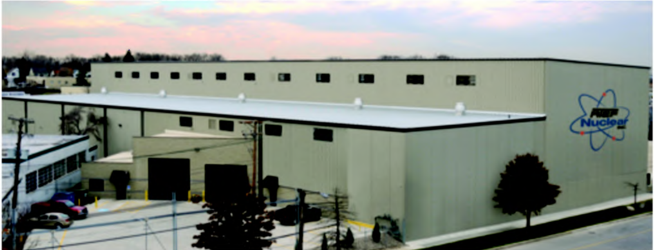
The AT&F Nuclear Fabrication Building in Cleveland, Ohio, offers clean-environment fabrication, welding, and assembly.
