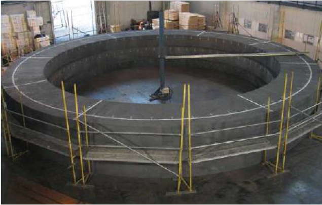
Figure 1.13 Test assembling of a blast furnace lining.
