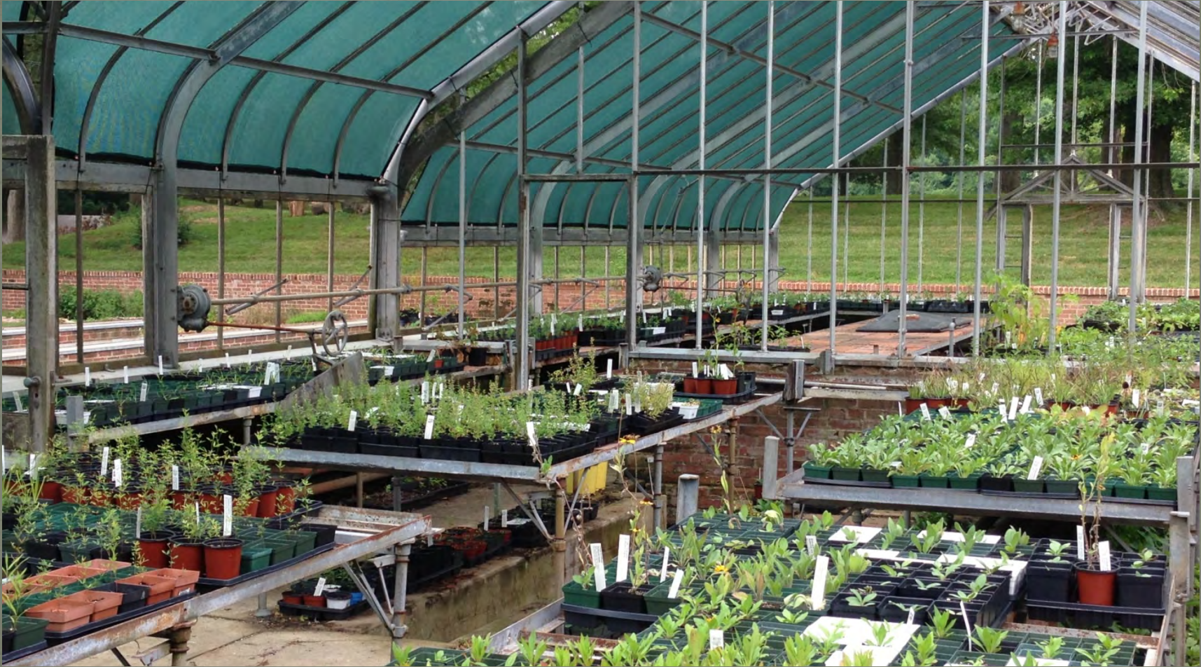
The historic 1935 Lutten Solar V-Bar greenhouse at Mount Airy Mansion, Rosaryville State Park
