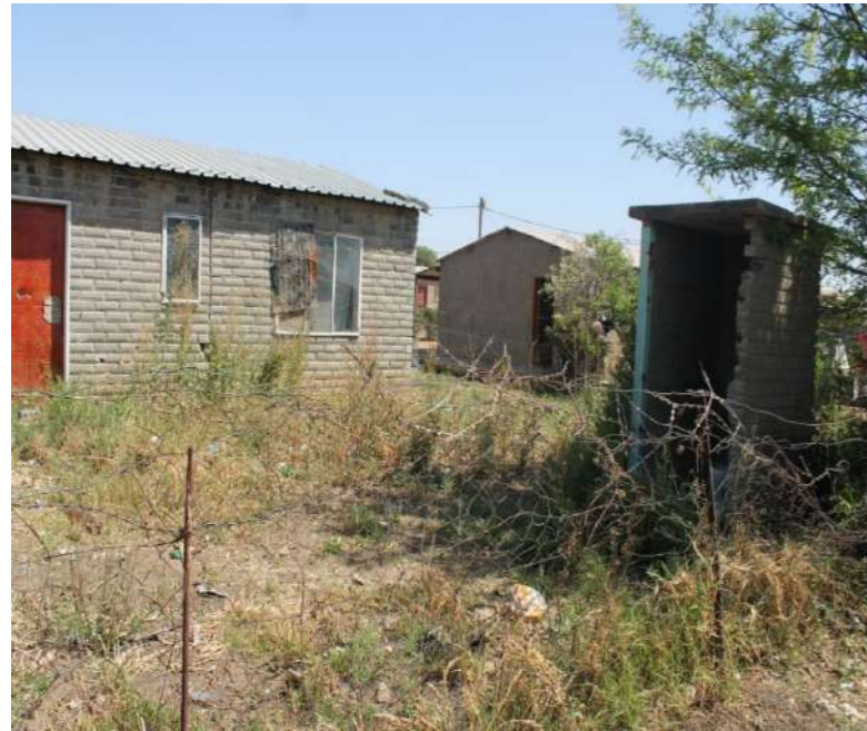
Figure 3: Overgrown grass on the premises.
