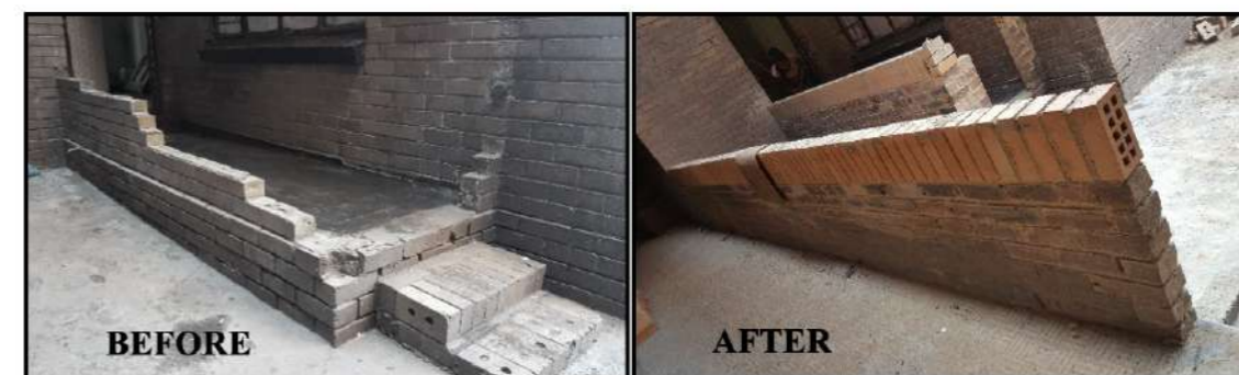
Figure 3: Before and after the repairs to the brick balustrades (Lamprecht, 2019).
