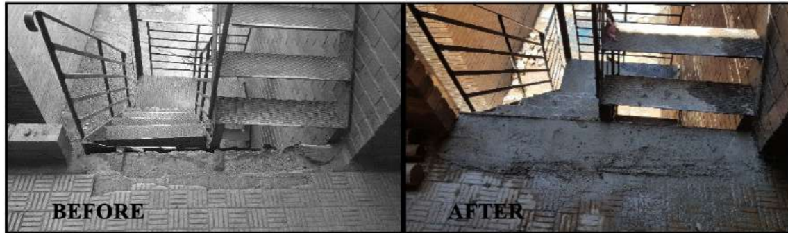
Figure 4: Before and after of the repairs to the steel staircase (Lamprecht, 2019).
