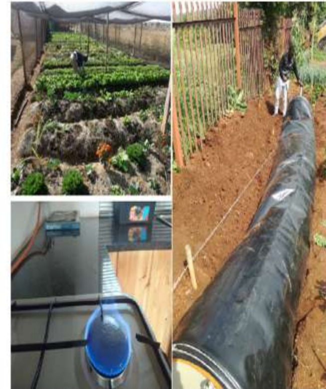
Figure 6: The food garden at a local school, a blue flame from the biogas stove at Siyakhana food garden and the installation of a plug flow biodigester
