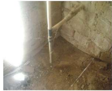
(e) digester with steam trap
