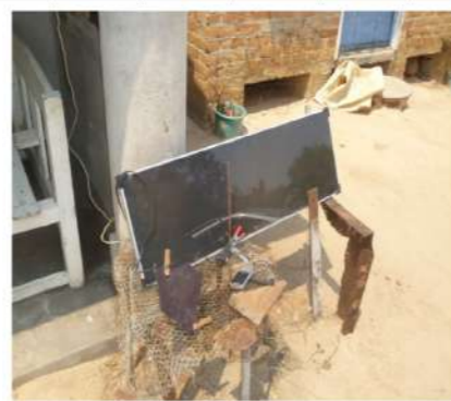
(b) Solar panel
