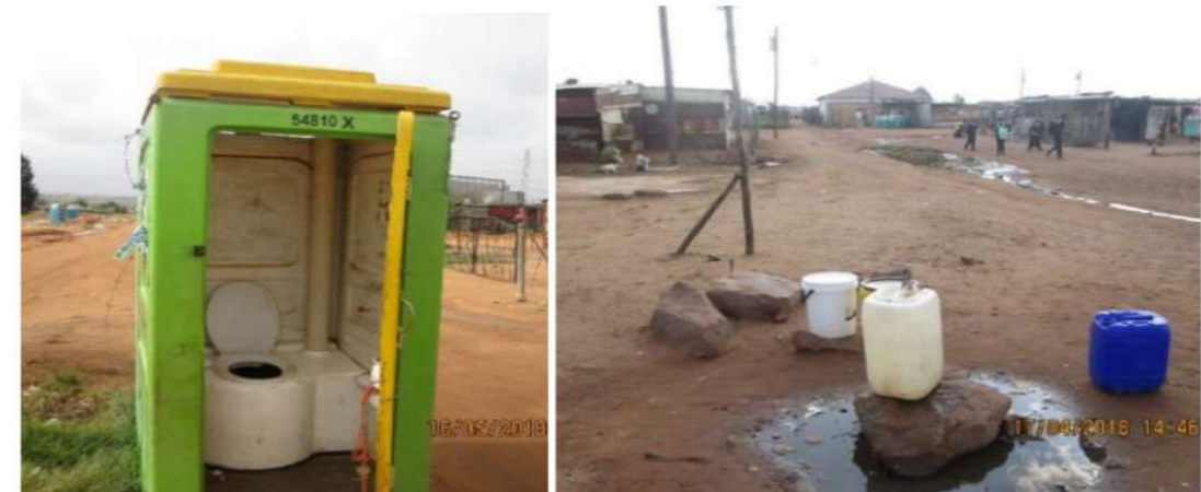
Figure 2. Chemical toilets (left) supplied in Zithobeni Extension 8 Informal Settlement and communal taps (right).
