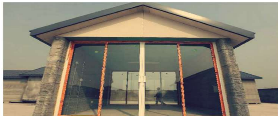
Figure 5: Winsun 3D concrete printed house (Winsun Decoration Design Engineering Co, 2015)
