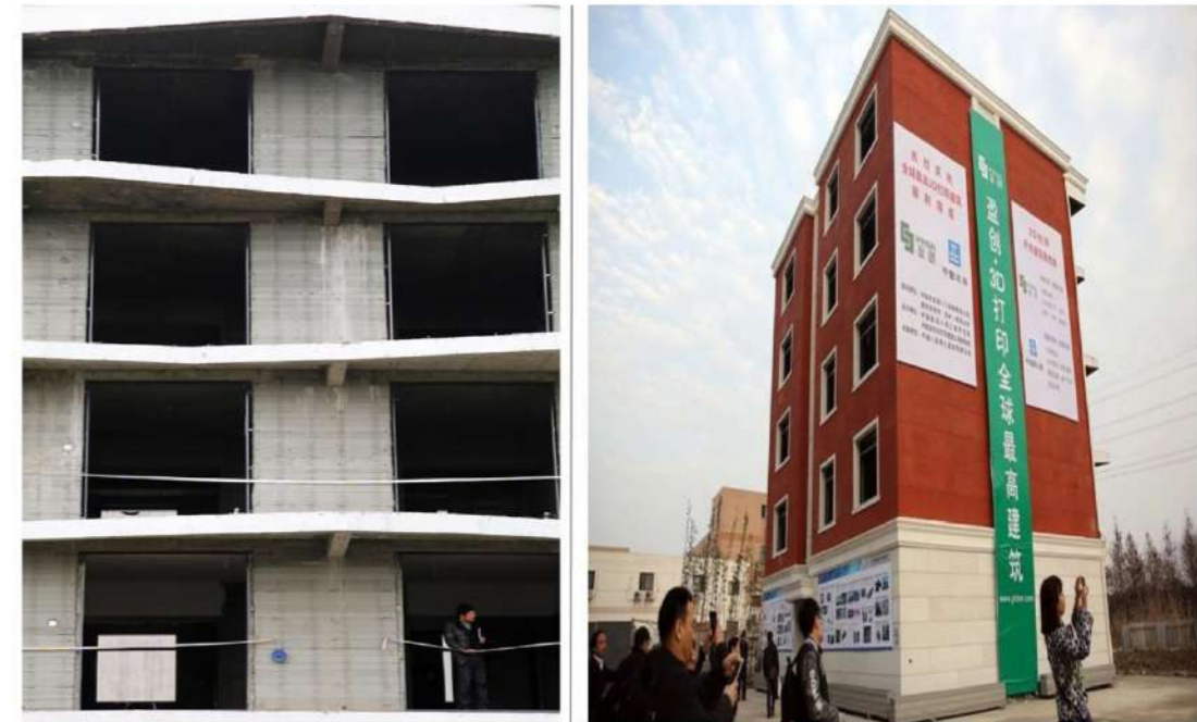
Figure 6: Winsun 3D concrete printed apartment block (Winsun Decoration Design Engineering Co, 2015)
