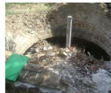
(a) abandoned digester
