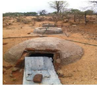
(f) abandoned digester
