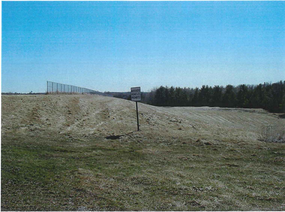
Northwest corner of landfill Looking south 4/3/06
