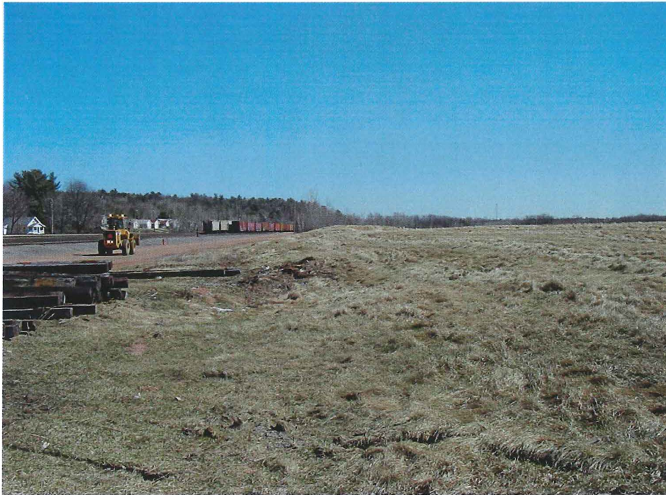
Northeast corner of landfill Looking south 4/3/06
