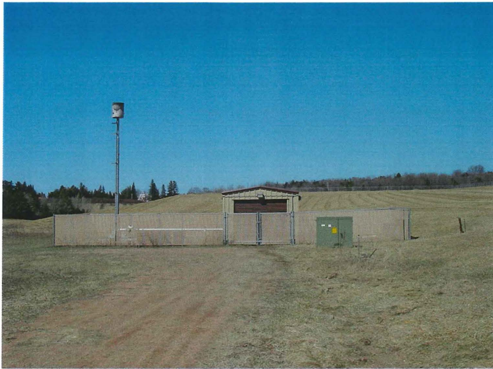
Blower Building Looking North 4/3/06
