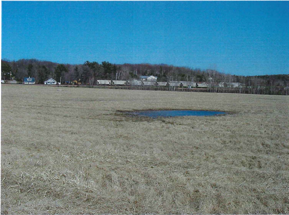
Water ponded on landfill cap Looking northeast (EW-3 in background) 4/3/06
