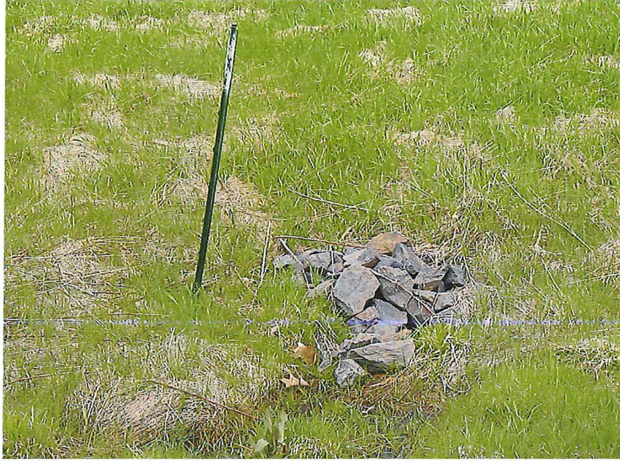
Toe drain on west side of landfill 05/01/2007
