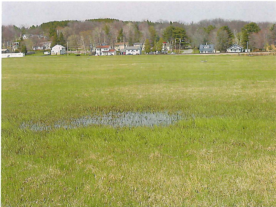
Ponded water on cap looking west north-west 05/01/2007
