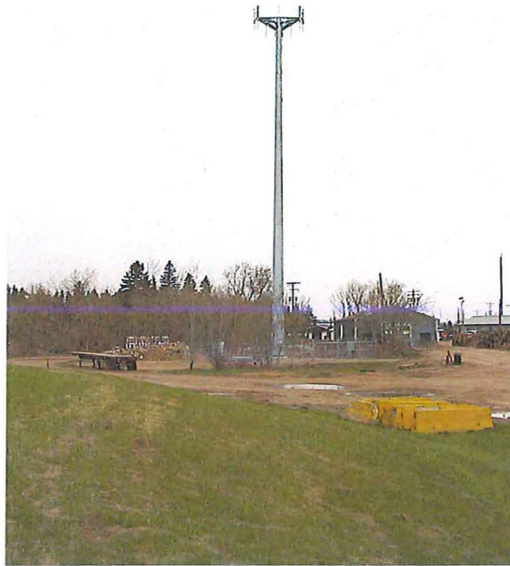
Antenna tower constructed on Holtz Krause property to north of landfill cap 05/01/2007
