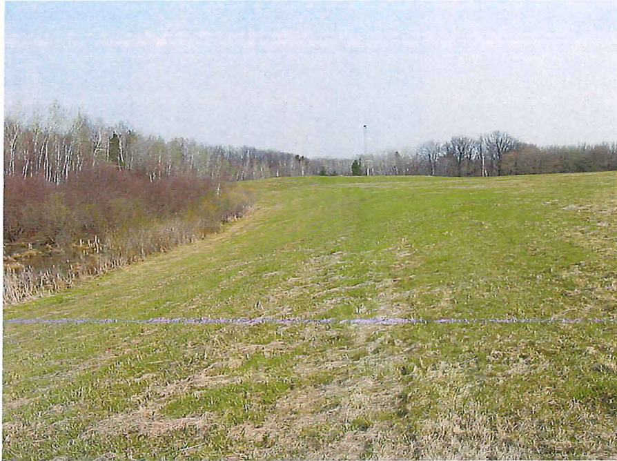
East bank of cap looking south 05/01/2007
