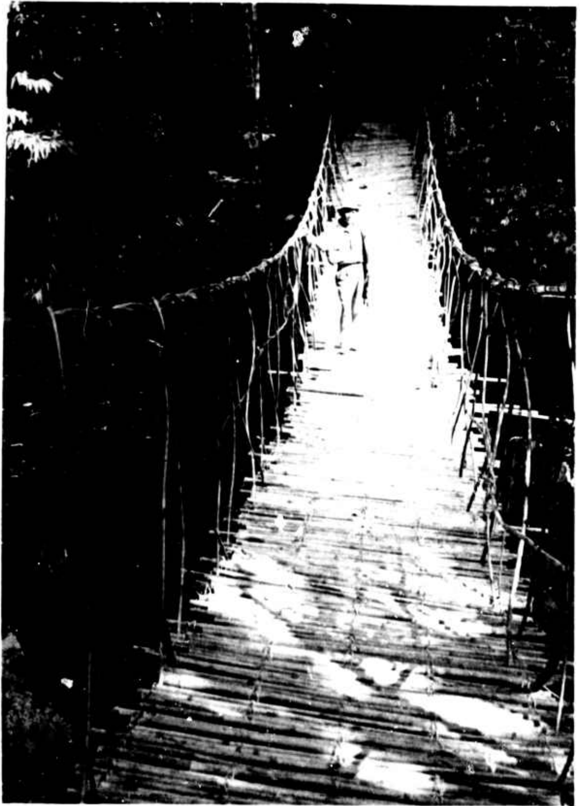
Fig. 19. Swing bridge made of bamboo (floor) and rattan (cables), Khao Yai National forest, central Thailand.
