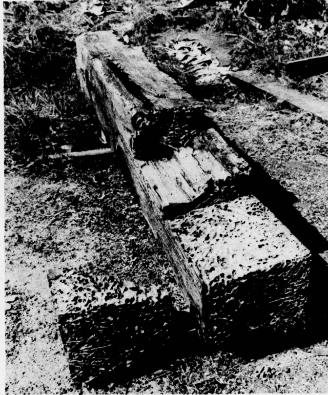
Fig. 3 — Fender timber thoroughly infested by marine borers. The outer surface gives little indication of the extent of internal damage.
