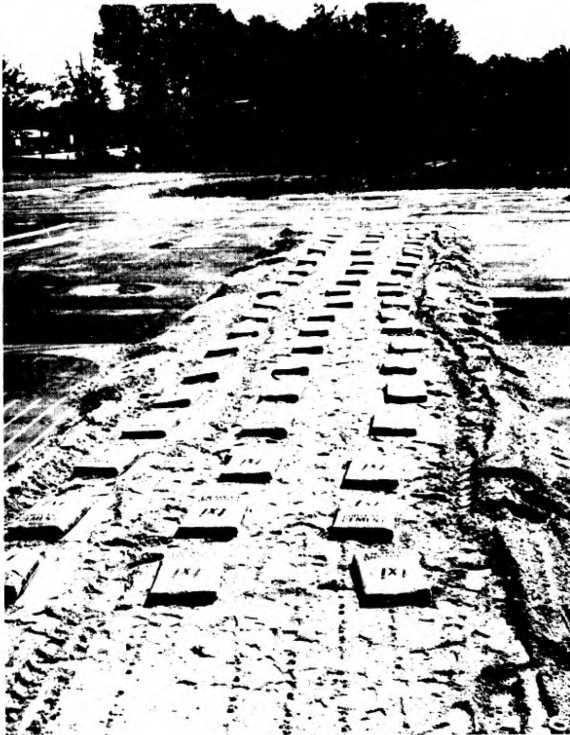
Figure 12. Portland Cement Distributed Over Sandy Gravel
