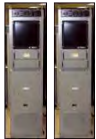
Two Redundant Launch Control Units
