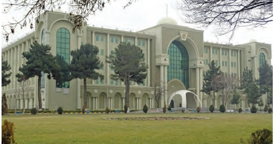
Afghan Ministry of Defense headquarters building in Kabul, January 7, 2016. (SIGAR photo by Wilhelmina Pierce)
