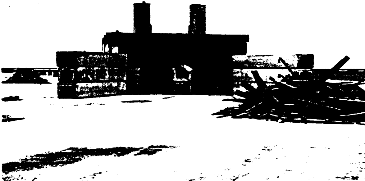
PLATE 22. INCINERATOR FOR WOOD DUNNAGE
