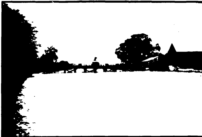
Photo No. 1. Looking downstream at temporary bridge used during construction of Union Road bridge during the flood of the summer of 1928.
