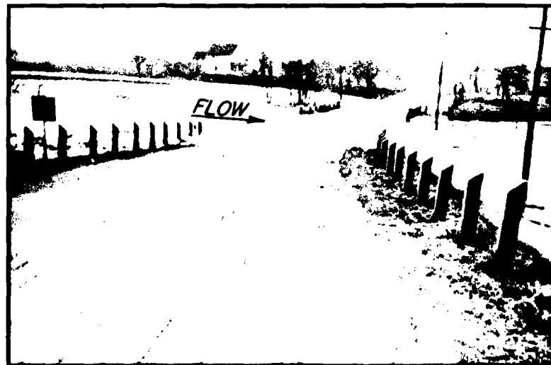
Photo No. 4. Looking south along Borden Road from bridge during the March 1942 flood.
