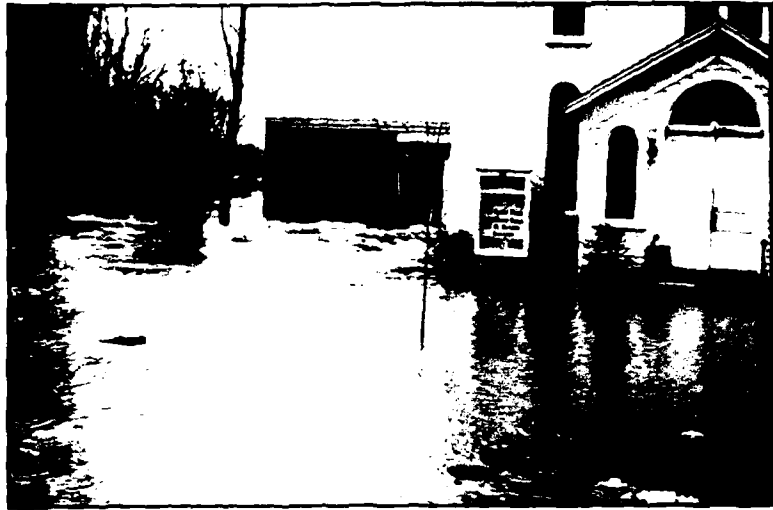
Photo No. 13. Elma Methodist Church and Sunday School addition on Bowen Road, during the March 1962 flood.
