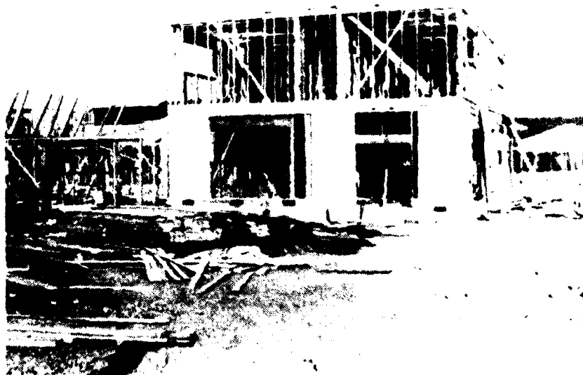
B) Typical Home Construction in Flood Plain Near Thomas Road and Princeville Street.
