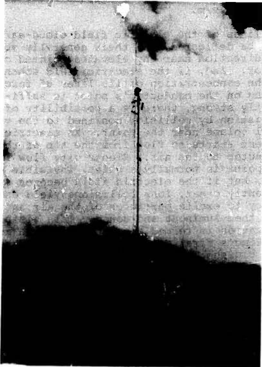
Figure 6, WBBH-TV Array, Ft. Myers, FL
