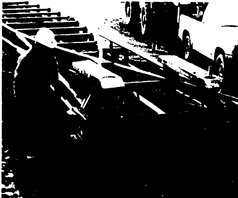
Business end of coring "fish." Drill rods exit the fish between spacer flanges, next to workman. Note lateral jacking pads which lock fish in place.
