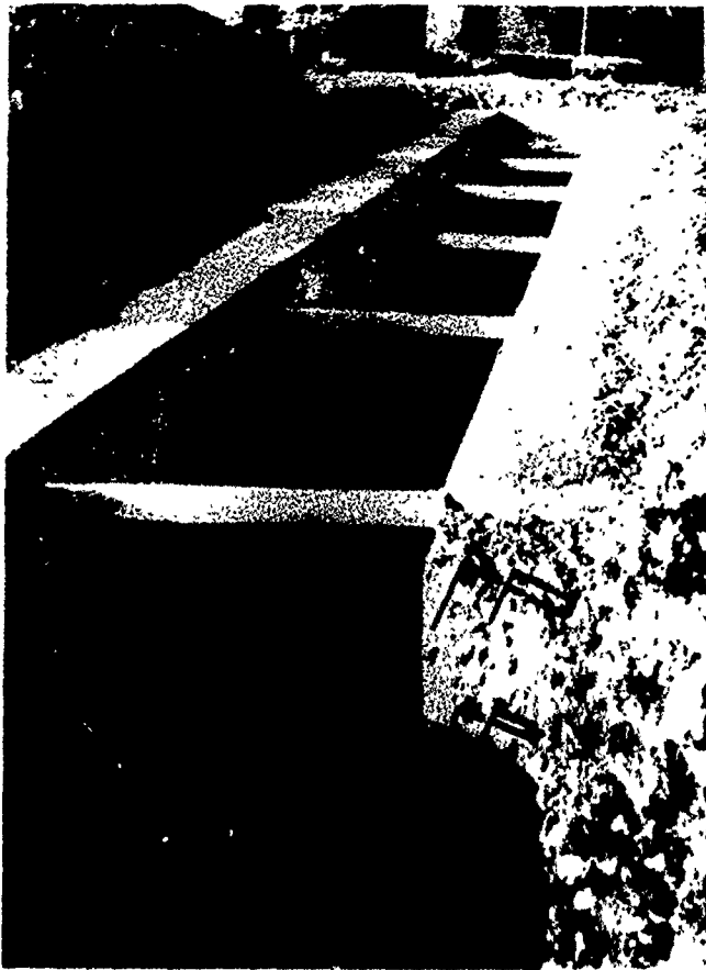
Typical construction of guide walls for hydrofraise.
