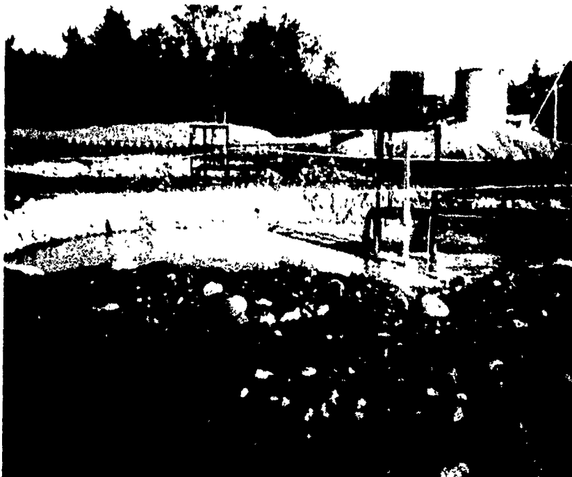
One of four bentonite slurry ponds. Note central pump and agitator. Concrete plant in background.
