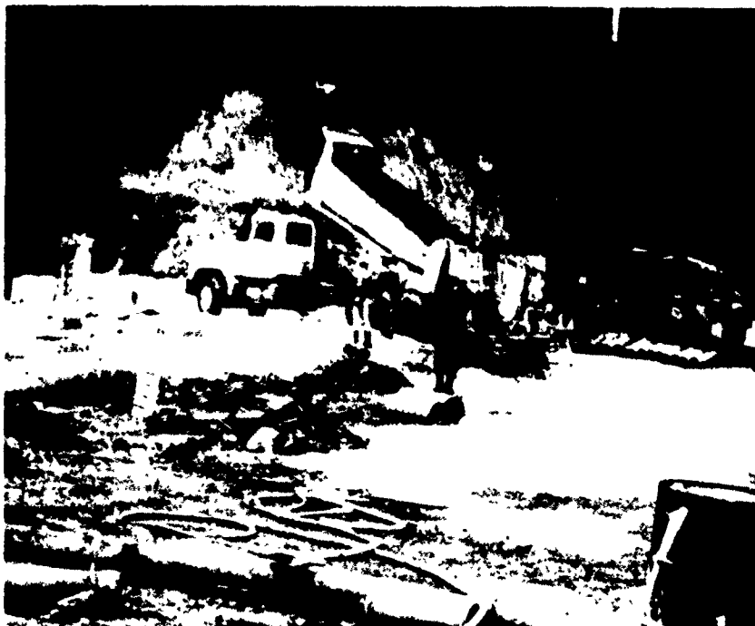
Emergency measures for uncontrolled slurry loss being implemented. Contractor is dumping wasted sand/silt mix from desander back into panel to help seal cracks.
