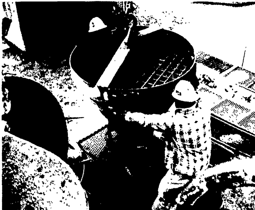
Unscrewing hopper from pipe coupling to prepare for the shortening of the tremie pipe length.
