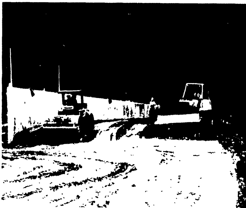
Backfill and compaction during dam raising. This strip either side of CIP wall was compacted with hand-operated tamper.
