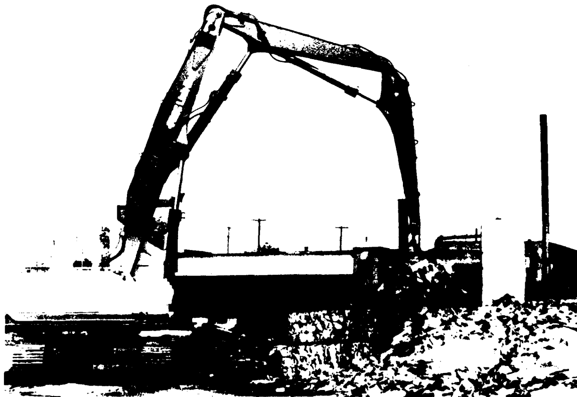
Figure III-9. Crawler mounted, hydraulic knuckle-boom crane with magnet.
