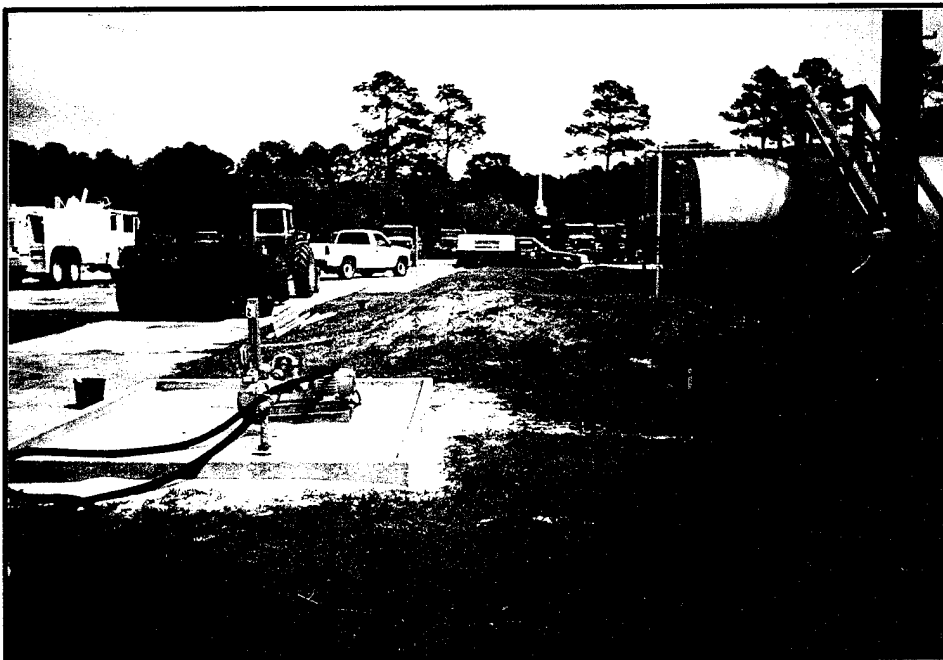
SITE 3: NORTHERN END OF ABOVE-GROUND FUEL STORAGE TANK AND BERM. THE BLUE TRUCK IN THE CENTER OF THE PHOTOGRAPH IS LOCATED ATOP THE ADJACENT UNDERGROUND FUEL STORAGE TANKS.
