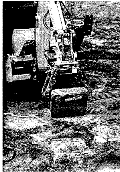
Figure 6: Gripper excavating M19 AT mine
