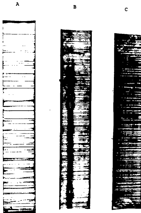
Figure 50. Different Forms of Damage Observed: (a) Dispersed Longitudinal Cracking and Transverse Cracking; (b) Localized Longitudinal Cracking and Delaminations; (c) Local Delamination at the Junction of Longitudinal and Transverse Cracks
