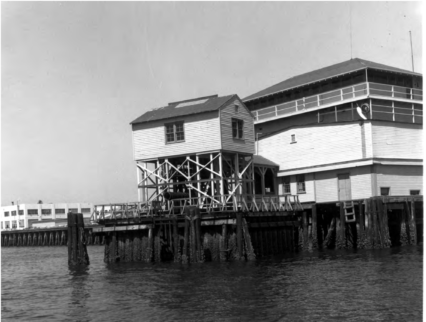
The Firing Tube and Submersible Elevator at Pier 1
