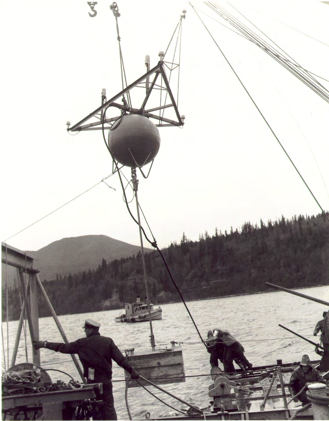
High Frequency Array Installation
