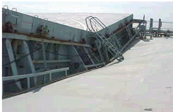
Figure 8 – Vacuum damage in way of a ballast hold
