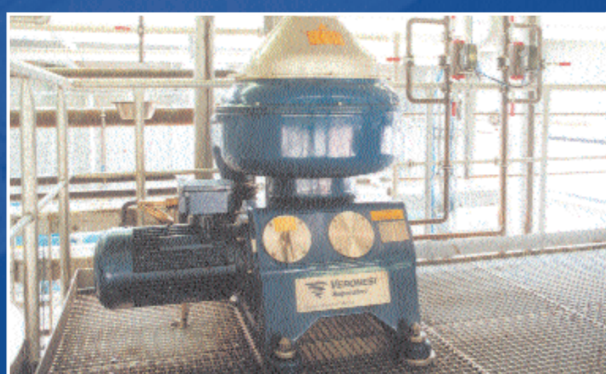
Final oil/water separation
