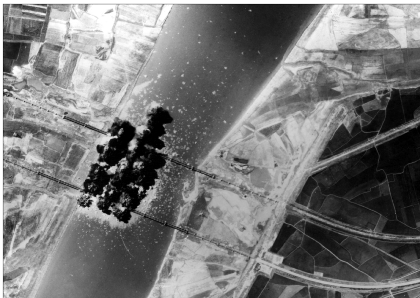
Bombs from FEAF Bomber Command B-29s smother a pair of railroad bridges north of P'yŏngyang on July 27.
