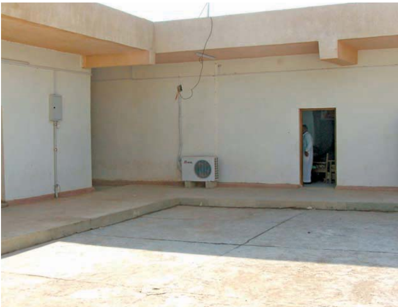
Sagrah School courtyard and split air-conditioning unit.
