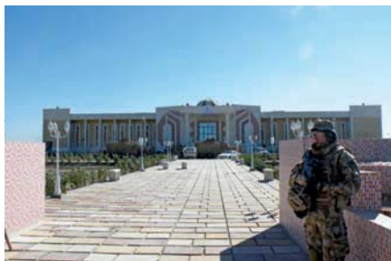
Sidewalk leading to the Basrah Courthouse and Witness Protection Facility.
