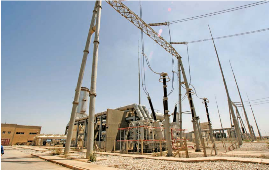
One of the RIE-funded projects to restore Iraq's infrastructure.
