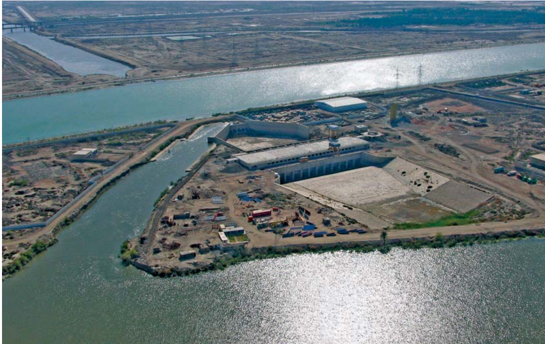
The Nassriya Drainage Pump Station, which is now complete, will help drainage in up to 220,000 hectares of farmland.
