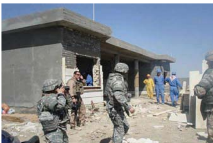
Al-Noor Primary Healthcare Center under construction. (OPA photo)
