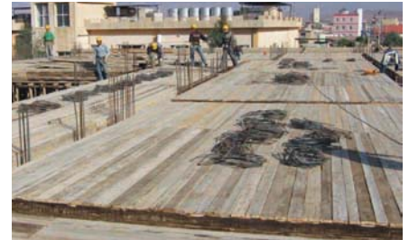
Construction of Emergency Hospital in Zakho City. (OPA photo)
