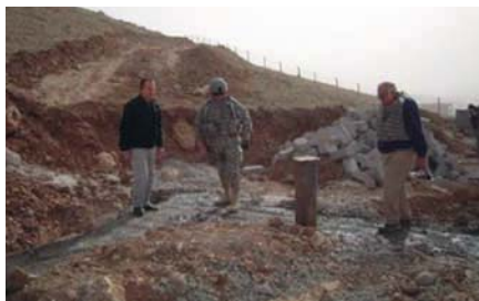
Construction of artesian water wells. (OPA photo)
