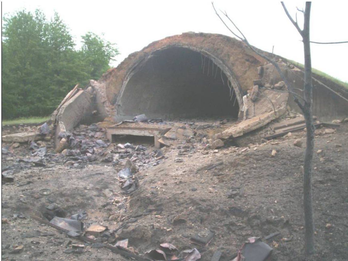
FIGURE 12. Earth-covered Magazine with Headwall Blown Out.
