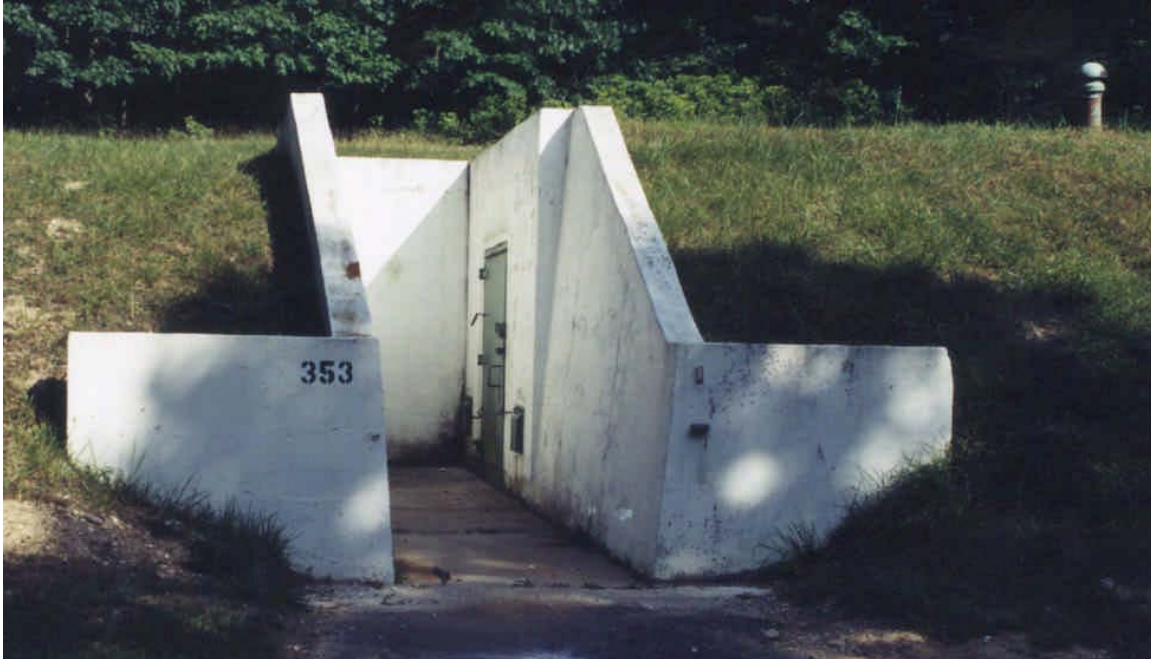
FIGURE 3. Magazine Similar in Design to One Destroyed at White Oak, Maryland, 28 June 1992.
