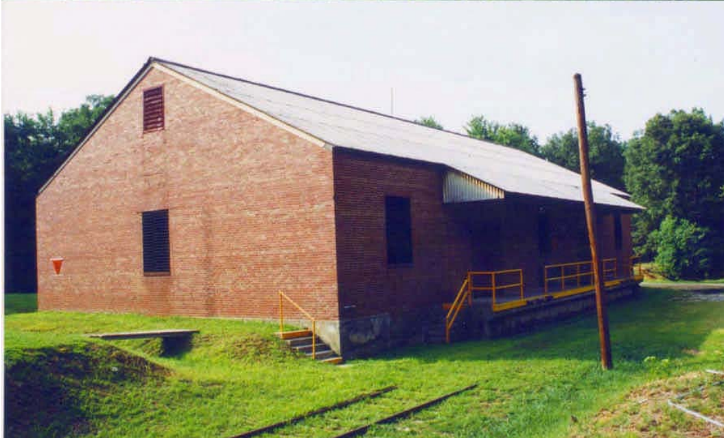
FIGURE 4. Magazines Similar in Construction to Magazine 518, Indian Head, Maryland.
