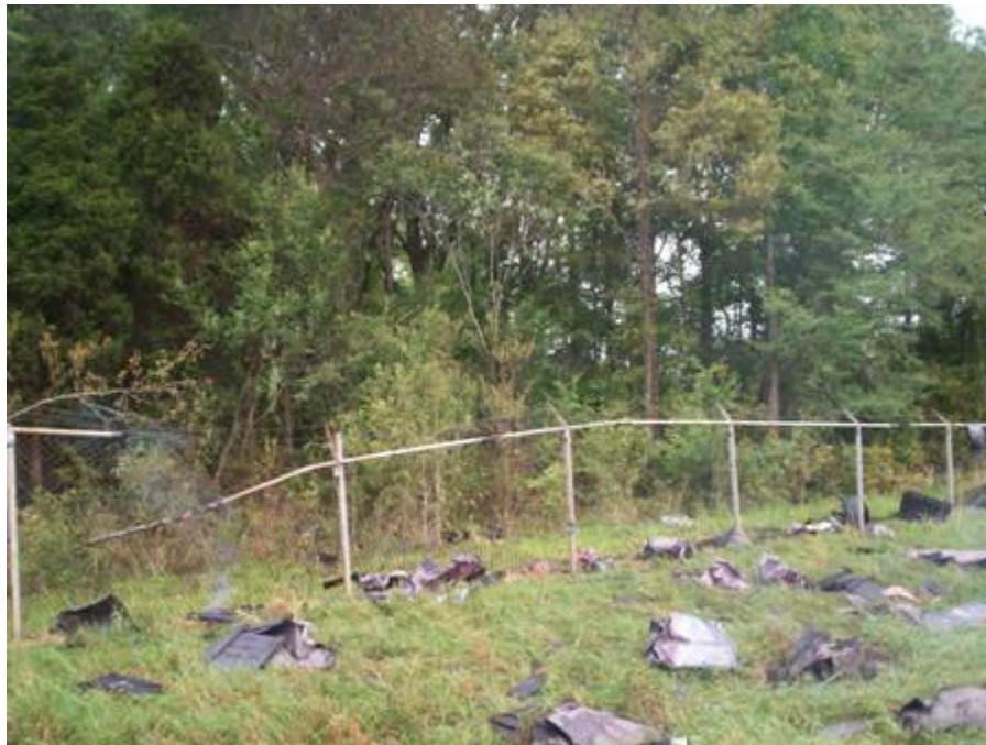
FIGURE 14. Debris Expelled from Magazine.
