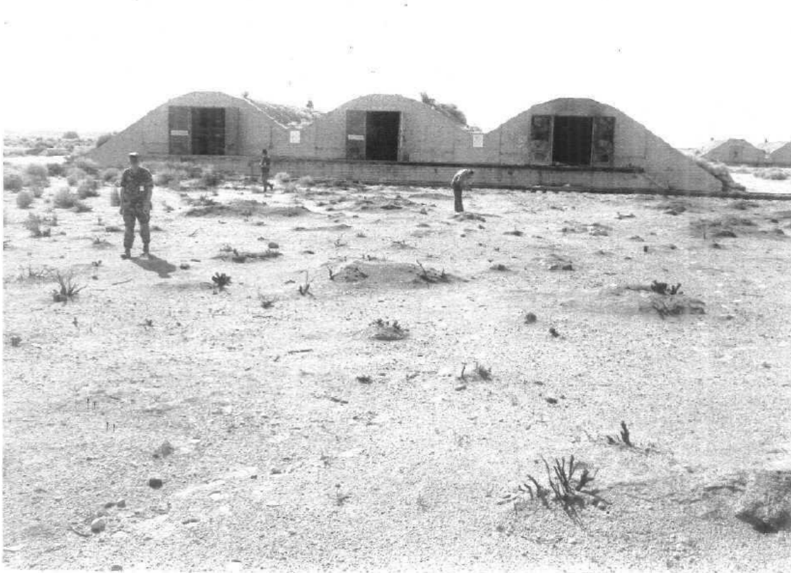
FIGURE 1. Three Arch Earth-Covered Magazine at Hawthorne Army Ammunition Plant. Fire occurred in unit on the right.
