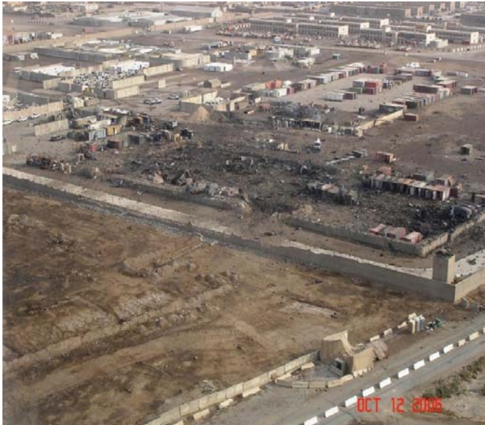
FIGURE 11. Damage at FOB Falcon near Baghdad, Iraq, 10 October 2006.
