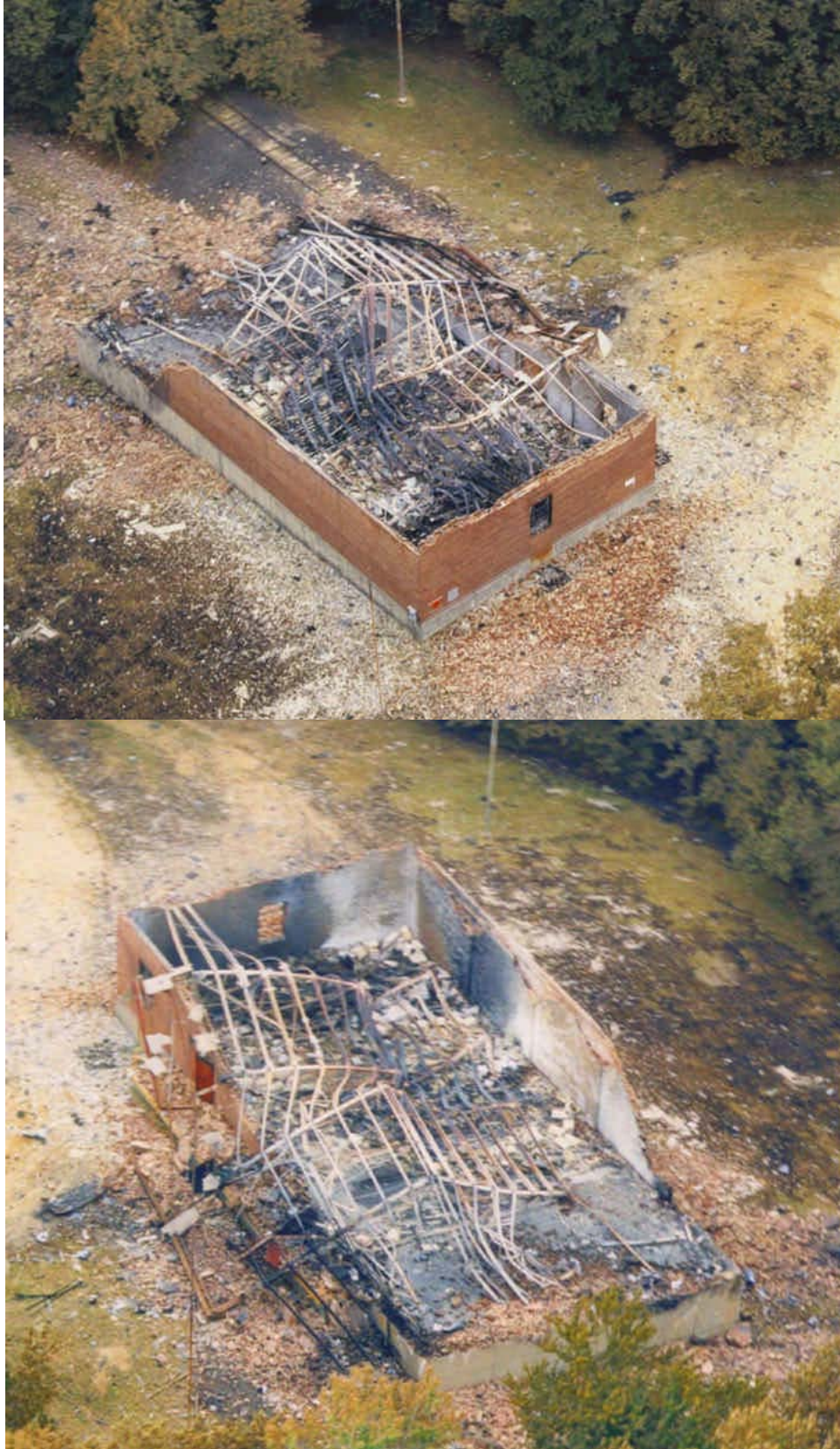
FIGURE 5. Magazine 518 after the Fires and Detonations.
