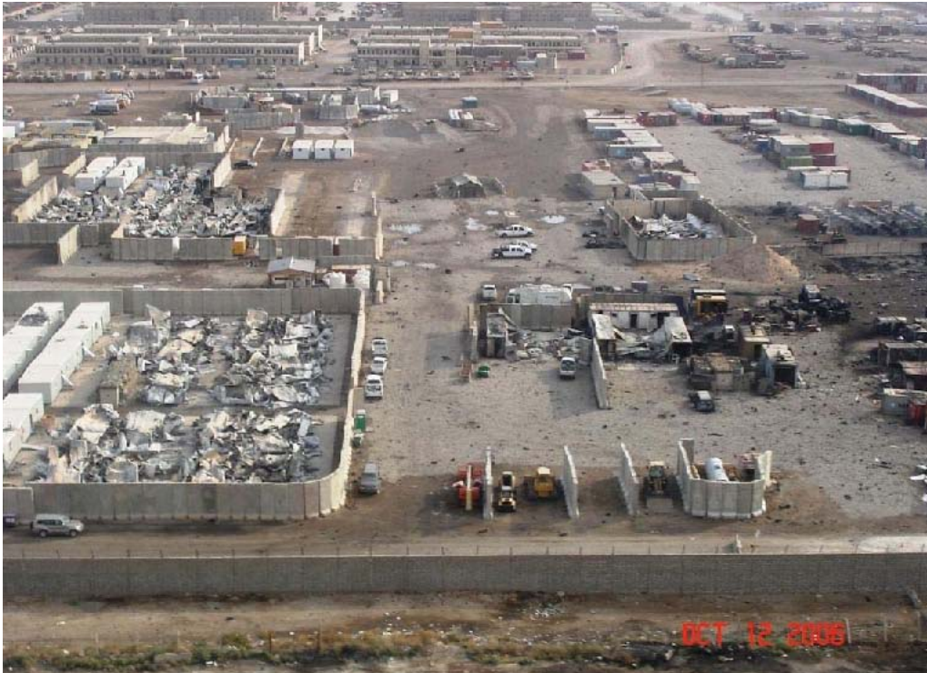
FIGURE 10. Damage at FOB Falcon near Baghdad, Iraq, 10 October 2006.
