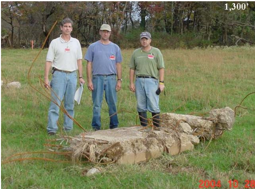
FIGURE 7. Large Fragment that had Been Part of the Headwall Found at Approximately 1,300 Feet from the Magazine.
