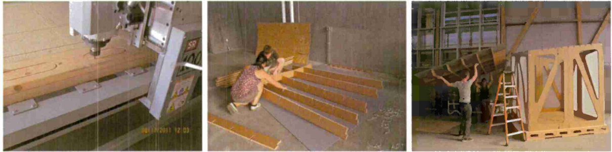
Figure 4: Digital fabrication techniques allowed the wood and cardboard elements to be quickly and precisely manufactured. Through design and fabrication advances, the structure became very light and easy to construct.
