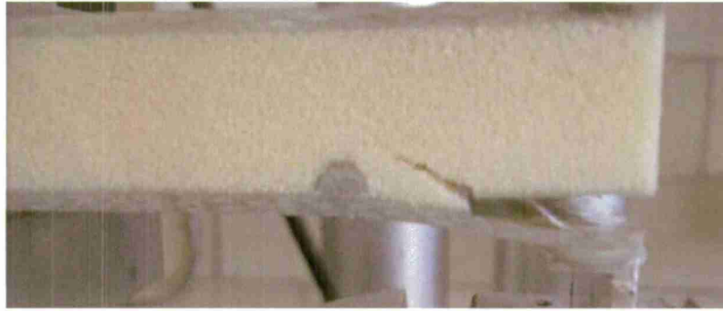
Figure 63 - Monotonic shear key failure due to cracks in foam
