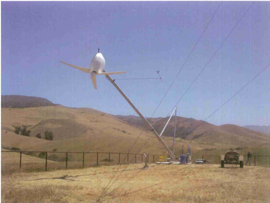
Figure 7: Wind turbine tower being raised. Due to the tower's "tilt-up" design, a cycle of lowering the tower, performing minor inspections or maintenance, and raising the tower again can usually be performed in under an hour.
