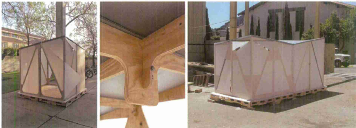
Figure 2: Views of earlier prototypes 3 (left) and 3X. These utilized plywood for the superstructure and resulted in more complexity and weight than desired; cardboard became the focus in prototype 4.
