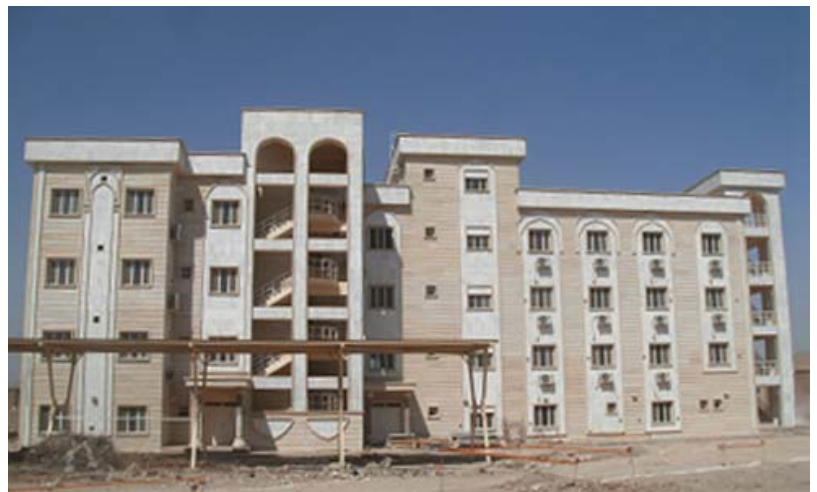
The $18.6 million project to build the Directorate of Counter-Terrorism is the only ongoing FMS project managed by USACE that is jointly funded by the GOI and the U.S. government. (USACE photo)
