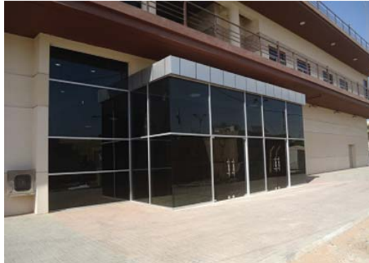
Construction of the ESF-funded Wazeriya National Training Center in Baghdad began in January 2011 and was expected to be completed in October 2012. (USACE photo)
