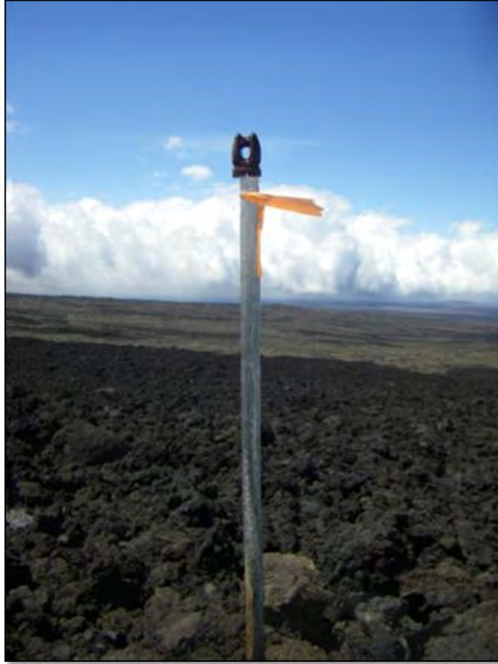
Figure 12. Example of a communication line pole with insulator – North view.
