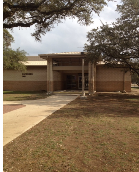
Photograph 2-3. The existing dining facility (Defender Inn) at JBSA-Camp Bullis
