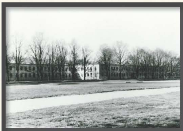
The magnitude of US Government's war-time functions demanded the construction of temporary buildings on the National Mall.
