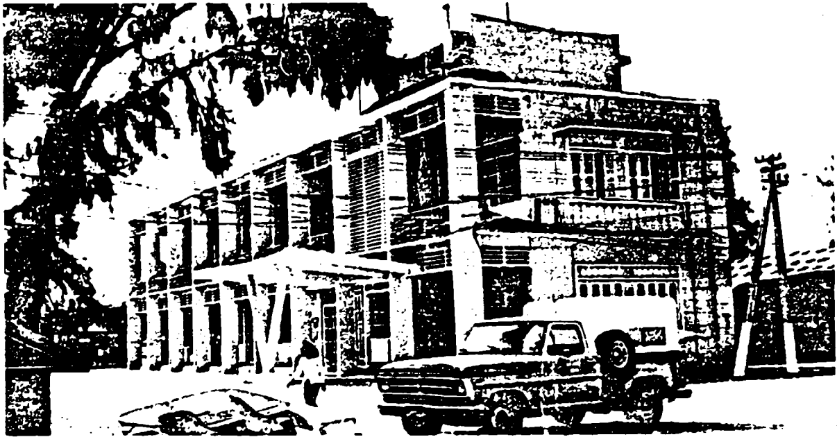
The ICCS Regional Headquarters in Da Nang.
