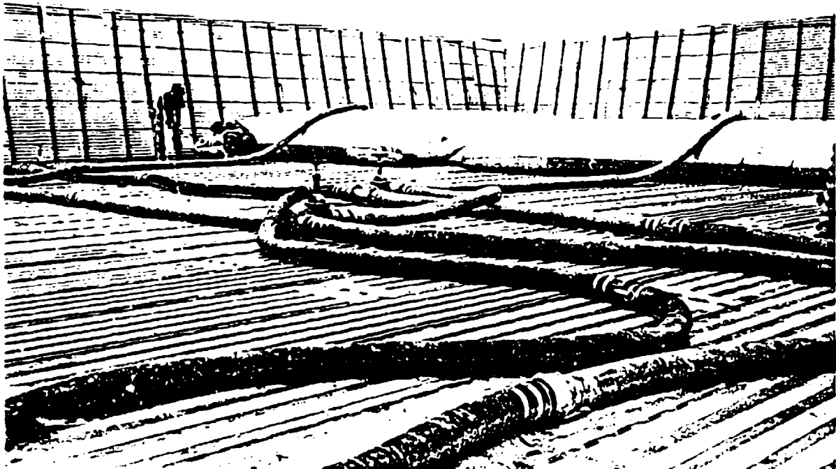
Installation of additional huge POL bladders was required to support the increased aircraft inventory.
