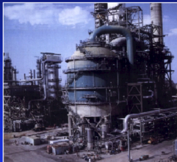
70 Ft Diameter Gasifier Unique Fluid Solids Processing
