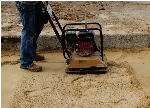
JPC-80 vibratory plate compactor.
