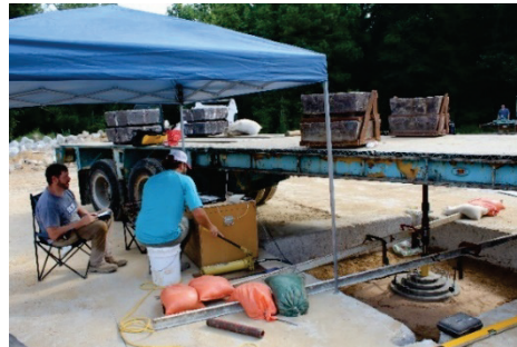
(a) Overall view of plate bearing test.
