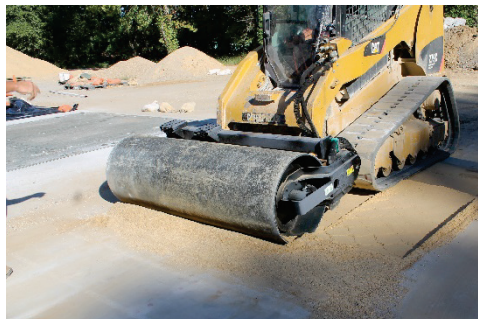
CAT CV18B vibratory drum compactor attachment.
