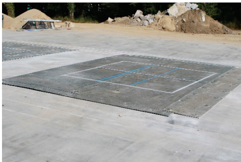
FRP panels assembled.
