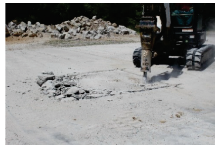
(b) Breaking withmoil-tipped hammer attachment on the mini-excavator.
