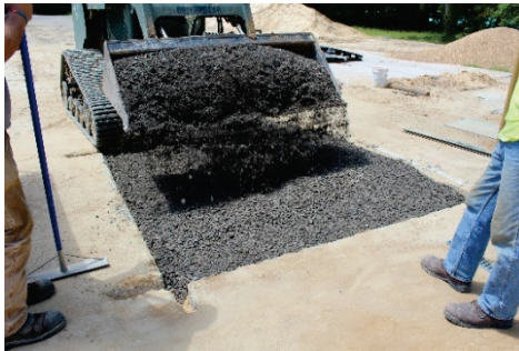
Placing GP-GM in repair.
