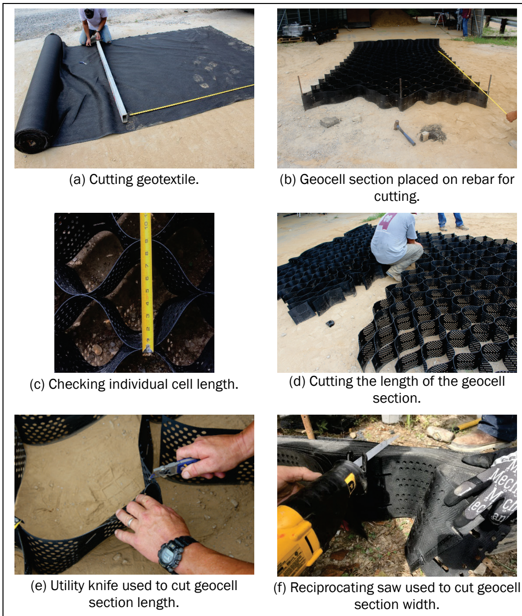
Figure 5-2. Cutting geotextile and geocell.
