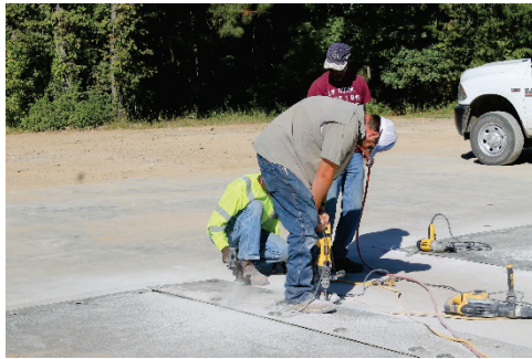
(c) Drilling through PCC.
