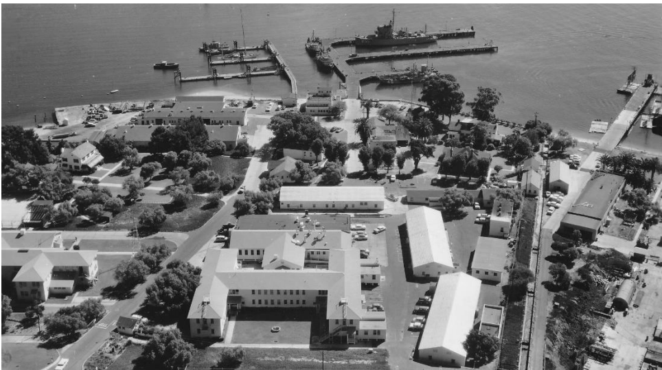
NELC Waterfront Area turned over to NUWC, which included only two major buildings, Bldg. 106 (foreground center) and 128 (left foreground), and Quarters L (left center).
