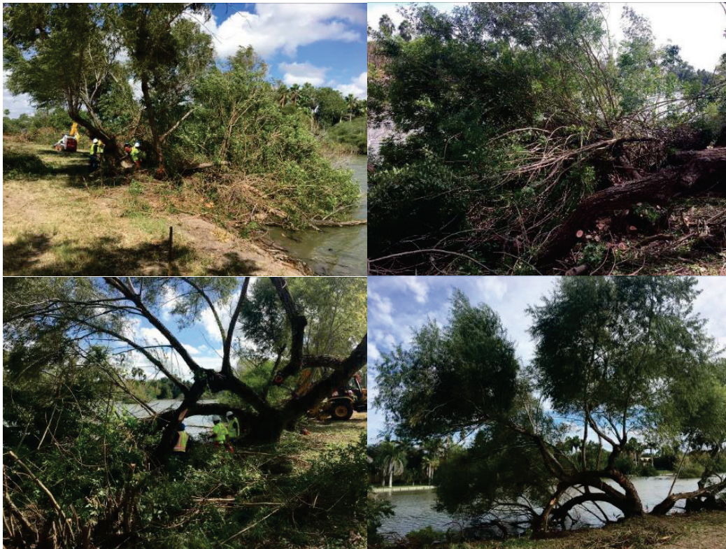
Figure B-5. Example of removing BPT around native vegetation (willows).
