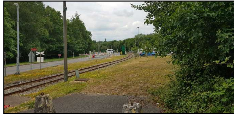
PHOTO E: VIEW FROM ACCESS ROAD NEAR PUBLIC RIGHT OF WAY
