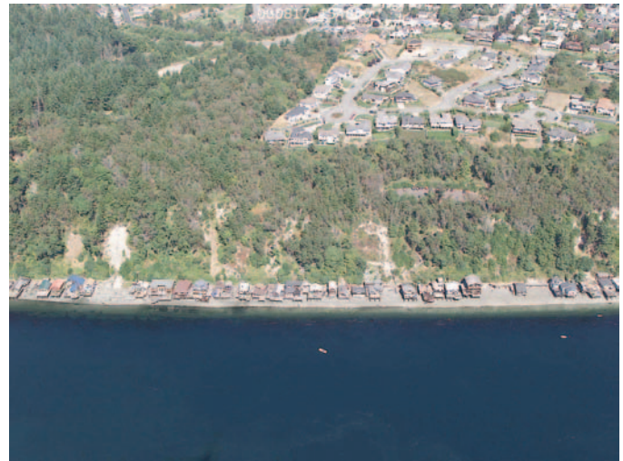
Figure 14. Salmon Beach community in Tacoma. Homes built over beach on piles at base of high bluff are periodically damaged or destroyed by landslides.
