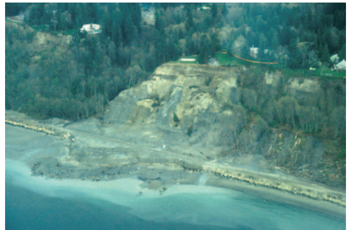
Figure 8. Large landslide north of Seattle that occurred in January 1997, following heavy rains. Note distinct mid-slope bench to the right of the landslide, marking the contact at the base of the glacial outwash. The landslide, which pushed a train into the Sound, involved a deeper failure in the underlying clay units. The toe of slope had been protected by the railroad grade at beach level for approximately 100 years and was not involved in the slide.
