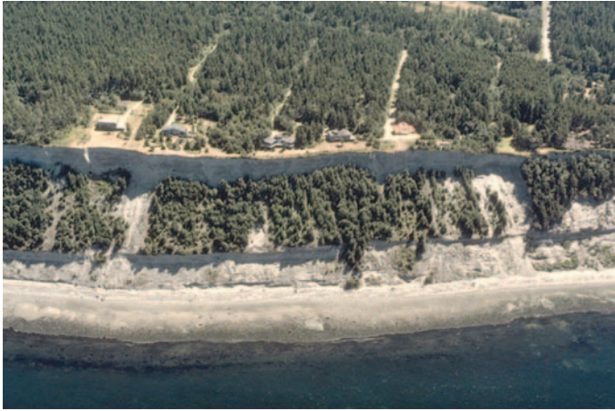
Figure 4. High bluffs near Port Townsend illustrate role of distinct stratigraphic units in defining bluff profile. Upper unit of glacial till fails in vertical slabs and does not support vegetation. Central sandier outwash unit is at angle of repose, with substantial revegetation between erosional events. Lower glacial unit is subject to wave action when storms and high tides coincide and when beach volume is reduced.
