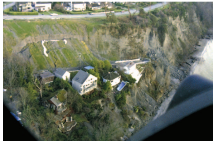
Figure 15. Homes destroyed by landsliding along Magnolia Bluff in Seattle during the winter of 1996-97. Homes had been built on a mid-slope bench formed by past erosion and landsliding.
