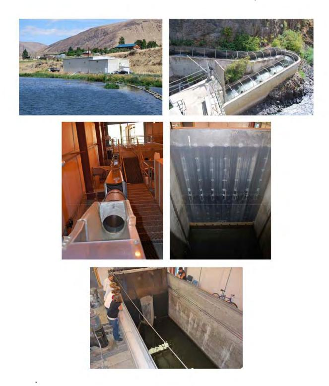
Figure 2-3. View of exterior of Roza adult fish collection facility (top left); pool and weir-type fish ladder (top right); fish chute to work area or back to river (middle left); fish lock (middle right); and adult holding tank (bottom, right).
