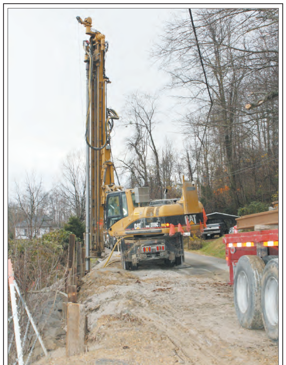
Workers were busy Wednesday morning repairing a major slip on Old Dixie Highway (Old U.S. 25). Crews had the road completely shut down. The slip is the second of four in the county that is being repaired primarily with FEMA funds. The first one repaired was on Mt. Zion Church Road. The final two to be repaired are on Buffalo Branch and Maret Cemetery roads.
