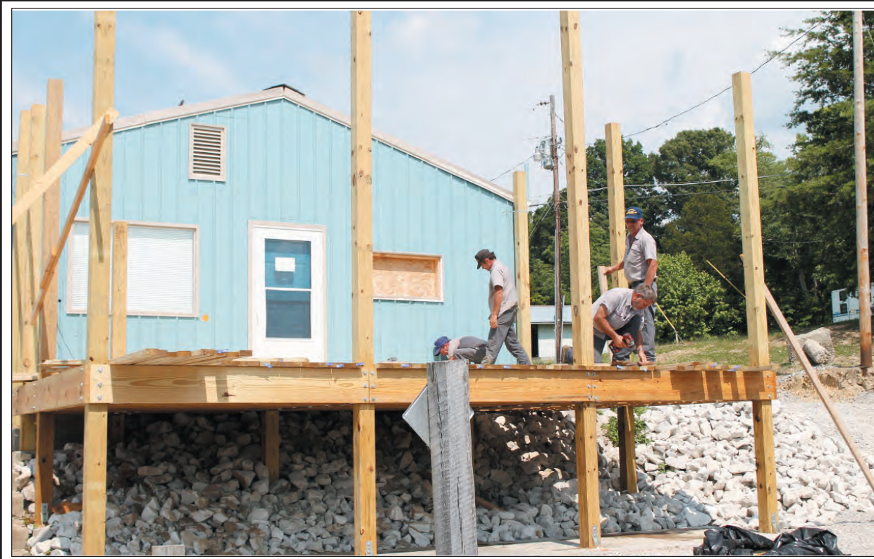
Mt. Vernon city workers are finishing up the new deck at the Lake Linville boat dock. The deck will include a dining area with an awning. The deck is scheduled to be completed before the Grand Re-opening of the boat dock next Wednesday.
