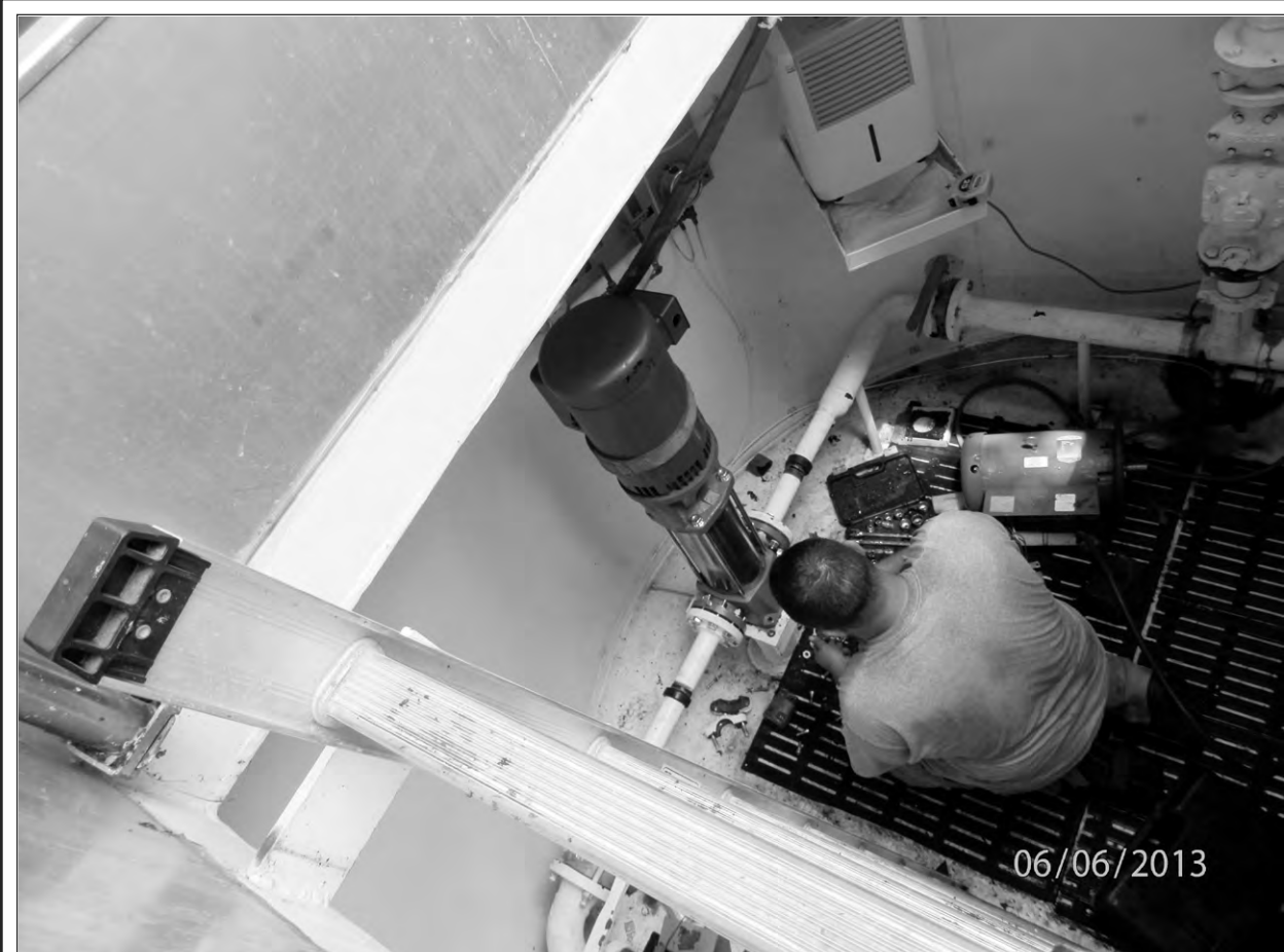
Eastern Rockcastle Water Association recently finished installing a new pump at their Sandhill pump station near Livingston. The motor quit on the old pump causing a new pump to have to be installed. The newly installed pump should prevent any interruption in service for the customer area, except during a power outage.
