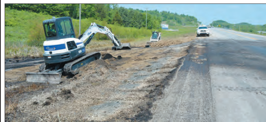
Workers from the Kentucky Transportation Cabinet spent over 24 hours cleaning and repairing the damage caused by a two vehicle accident Sunday on Highway 150 after a fuel truck, which had collided with a car, overturned, spilled fuel, burst into flames and melted blacktop. Crews opened the roadway after about 10 hours but are still working to clean up the fuel that spilled into the ground around the accident.
