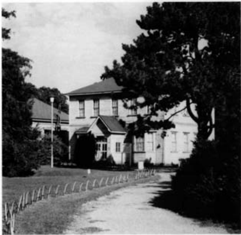
The Administration Building of the Botanic Garden of Hokkaido University in Sapporo. The architecture shows the influence of Dr. William S. Clark, a New Englander who helped develop the garden. (All photos are by author.)
