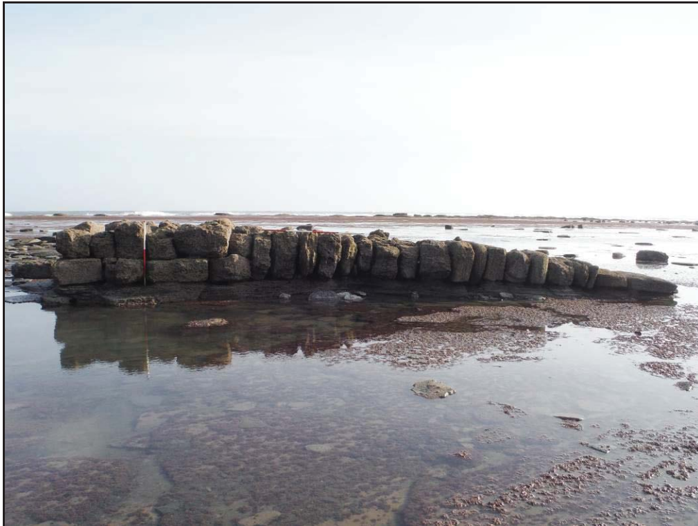
Figure 28- East facing view of the slipway at Saltwick (Scale- 1 x 1m & 1 x 2m)
