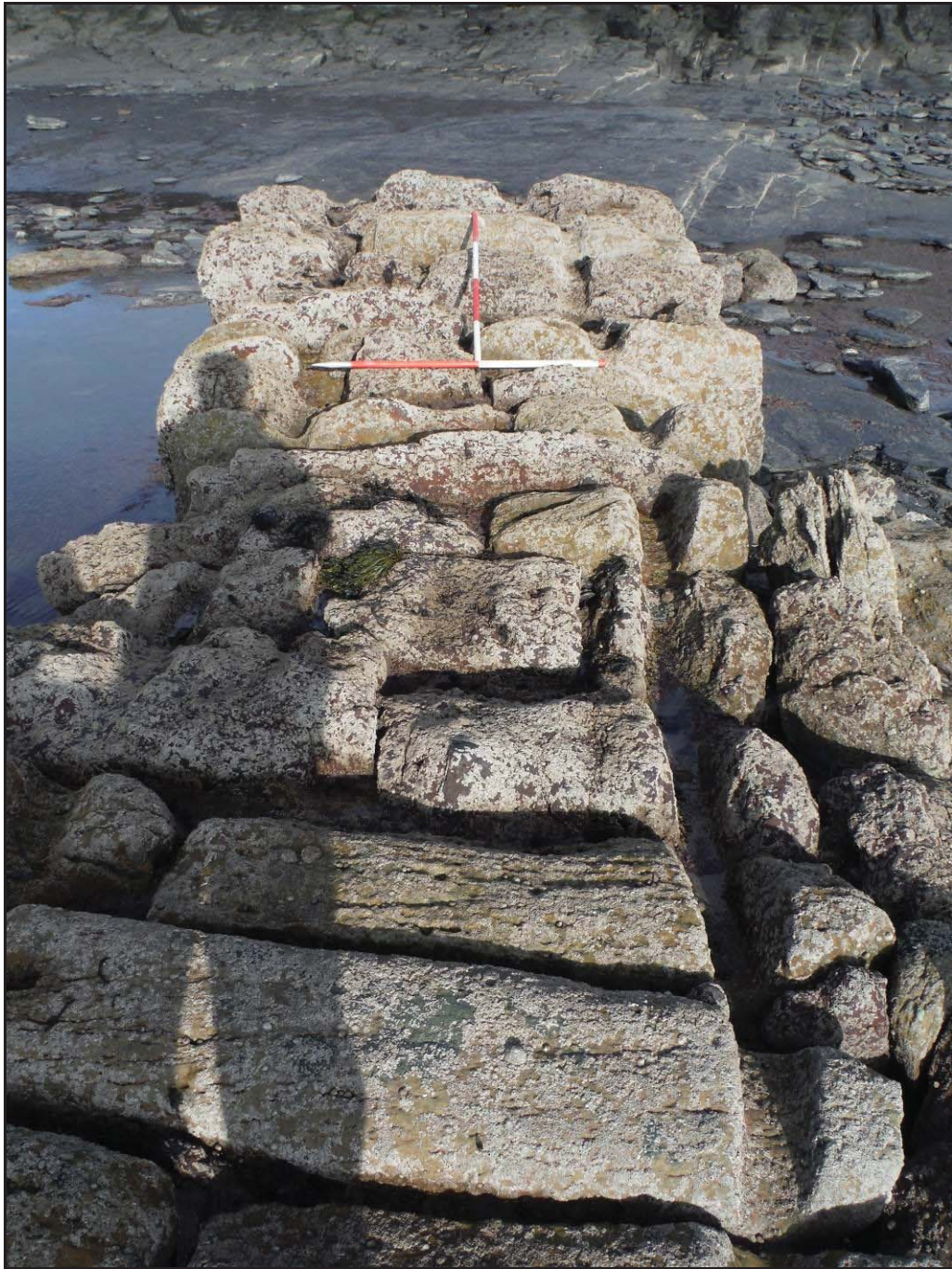
Figure 30 –NNW facing view of the slipway at Saltwick displaying the grooves/tracks cut into the superior surface of the stonework. (Scale- 1 x 1m & 1 x 2m).
