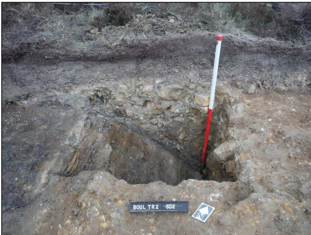
Figure 11- Building platform levelling deposits (205) and (204) associated with quarry dross [221]. (Scale- 1 x 1m)
