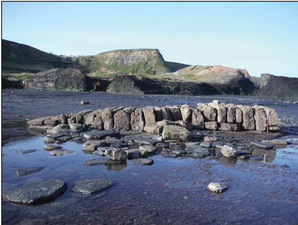
Figure 27- West facing view of the slipway at Saltwick (Scale- 1 x 1m & 1 x 2m)
