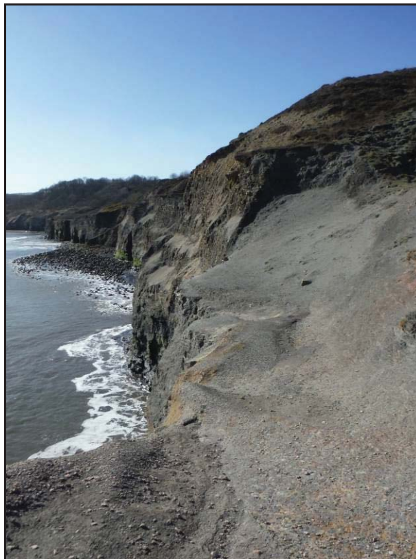
Figure 79- Continuation of the liquor channel eroded to the south of the steeping pits, looking south.
