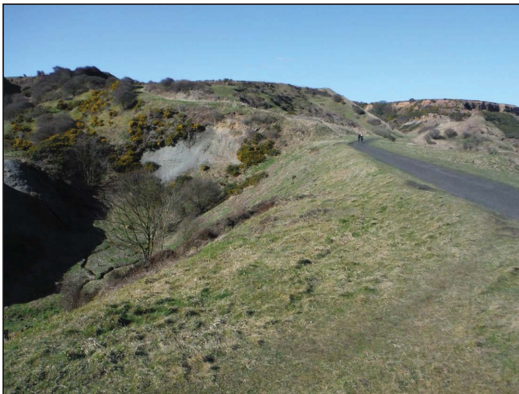
Figure 86- The large-scale railway embankment within Deep Grove Quarry, looking north-west.
