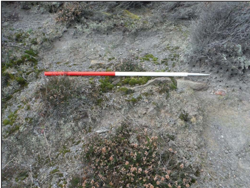
Figure 46- Remains of a stone retaining wall on the eastern face of the southern 'arm' of the lower quarry area, looking west (Scale- 1 x 1m).
