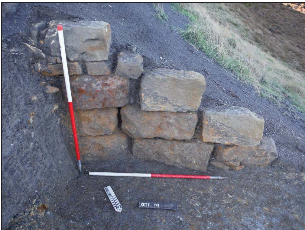
Figure 16- SW-facing view of retaining wall (103) (Scale- 2 x 1m)
