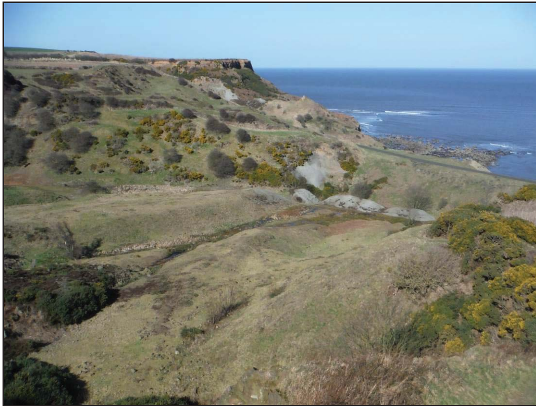
Figure 87- The south-western two-thirds of the quarry floor at Deep Grove, occupied by large spoil heaps, looking north. Note also the central water channel feeding in to a roughly triangular reservoir defined by the prominent bank of material along its north-eastern edge.
