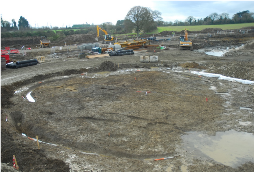
Post-excitation view of the penannular enclosure, looking southwest (top)
