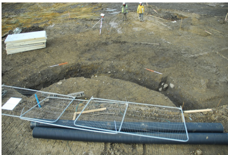
Post-excitation view of the barrow, looking east (top)
