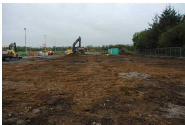
Monitoring in Field 2
