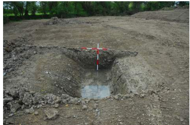
Mid-ex view of Ditch C11, looking south (top)
