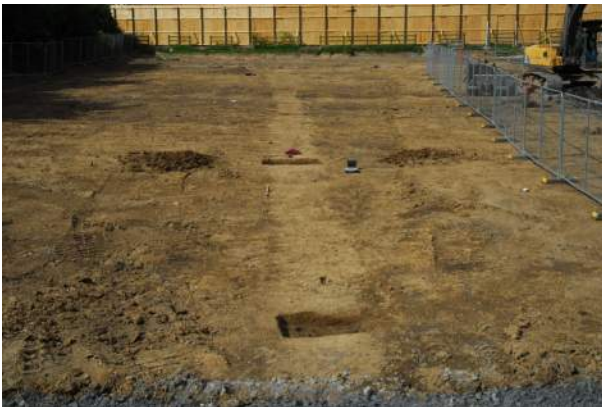
Mid-ex view of Ditch C6, looking north (top left)
