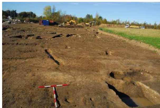
Mid-ex view of pit C601 truncated by slot trench C402, looking north (top)
