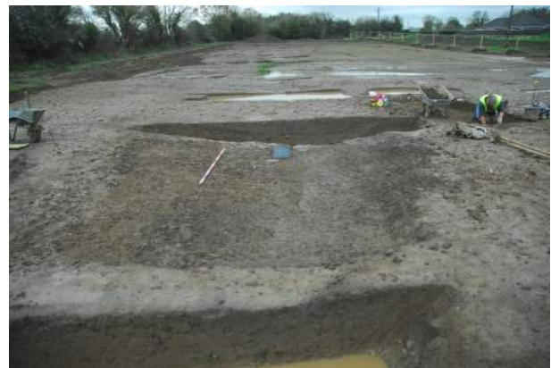
Mid-ex view of metallised surface C2334 crossing Ditch recut C2208, looking north (top)
