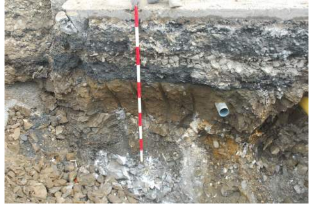
Working shot of service trench excavated across Drumree Road, with ditch C503 surviving in section below road gravels, truncated by a water pipe to the right (top)
